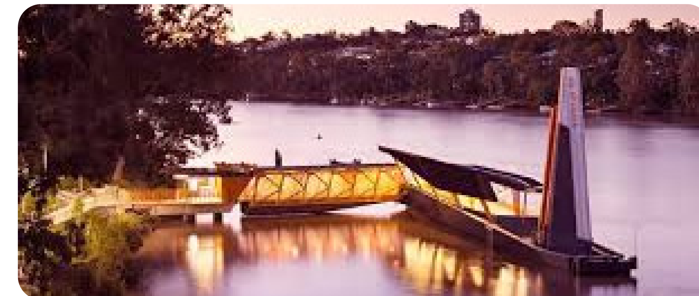
Brisbane Ferry Terminal - Queensland
